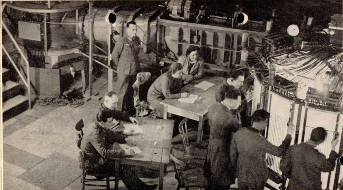
German scientific personnel work on German supersonic wind tunnel at Naval Ordnance Laboratory, Washington, D. C. Originally used at Peenemunde in V-2 development, the tunnel was captured by Americans in south Germany. At right, crew read data from bank of 120 manometers. Main valve at upper left.
