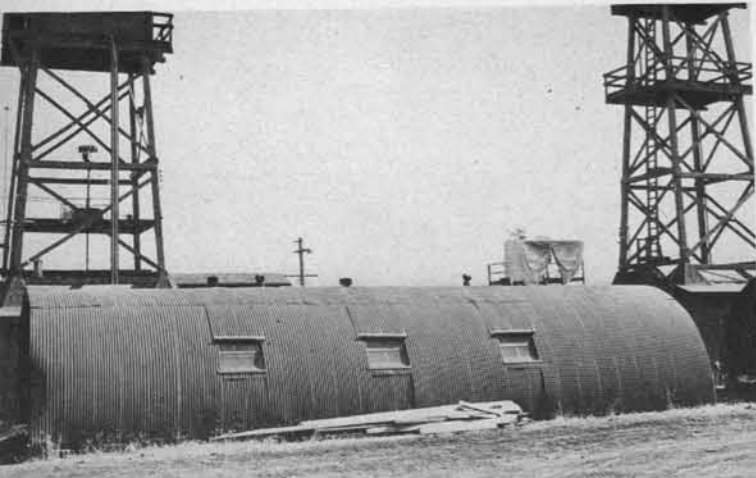
RPD project at Pacific Fleet Radar Center, now serving the fleet.
